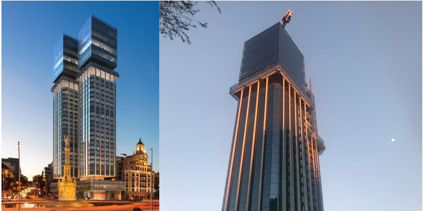
Cólon Towers rehabilitation
